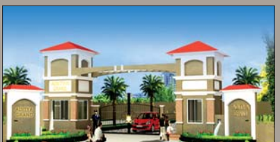
Aditya Grand - 50acres Mega Township Location: Visakhapatnam VUDA L.P No. 88/2015
